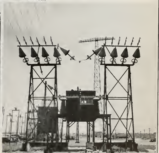
POWERFUL TRANSMITTERS ARE CONNECTED WITH THE ANTENNAS THROUGH LINES THAT ARE SHIELDED TO PREVENT SIGNAL LOSS.
