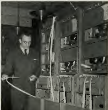
HOW THE HANDLING OF RADIOTELEGRAPH TRAFFIC WILL BE SIMPLIFIED UNDER THE PANDORA PLAN IS PICTURED BELOW. AT LEFT IS A TYPICAL MORSE UNIT WITH OPERATORS FEEDING PERFORATED MESSAGE TAPES INTO INSTRUMENTS LEADING TO AUTOMATIC PRINTERS. AT RIGHT, A ROW OF MODERN "PACKAGE SETS," EACH OF WHICH PROVIDES COMPLETE FACILITIES FOR THE TAPE-RELAYING OPERATIONS OF A CHANNEL.
